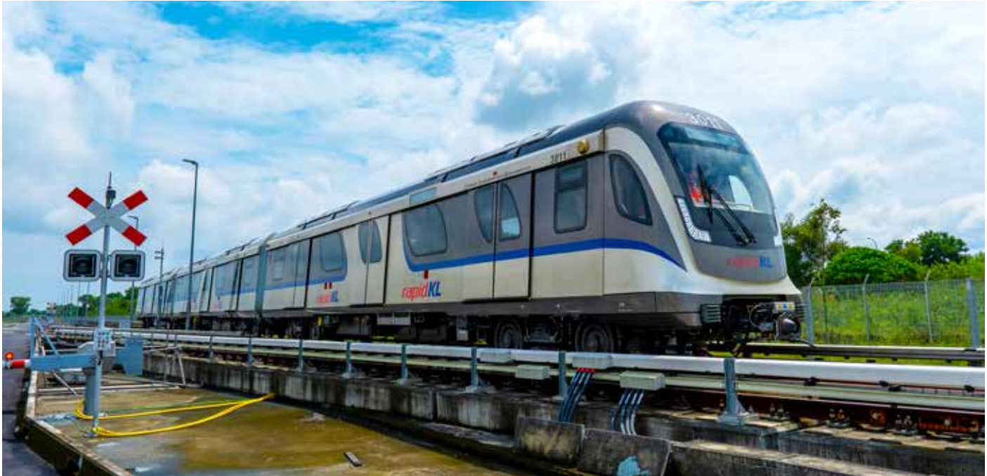
The Light Rail Transit 3 (LRT3) project, a significant infrastructure development project in our portfolio, achieved notable milestones in 2023. Almost all of the civil works were completed, achieving overall physical construction completion of 92% and financial progress of 88% at the end of 2023
